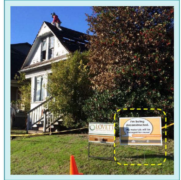
Example of mandated signage for deconstruction projects. Credit: City of Portland Bureau of Planning and Sustainability
